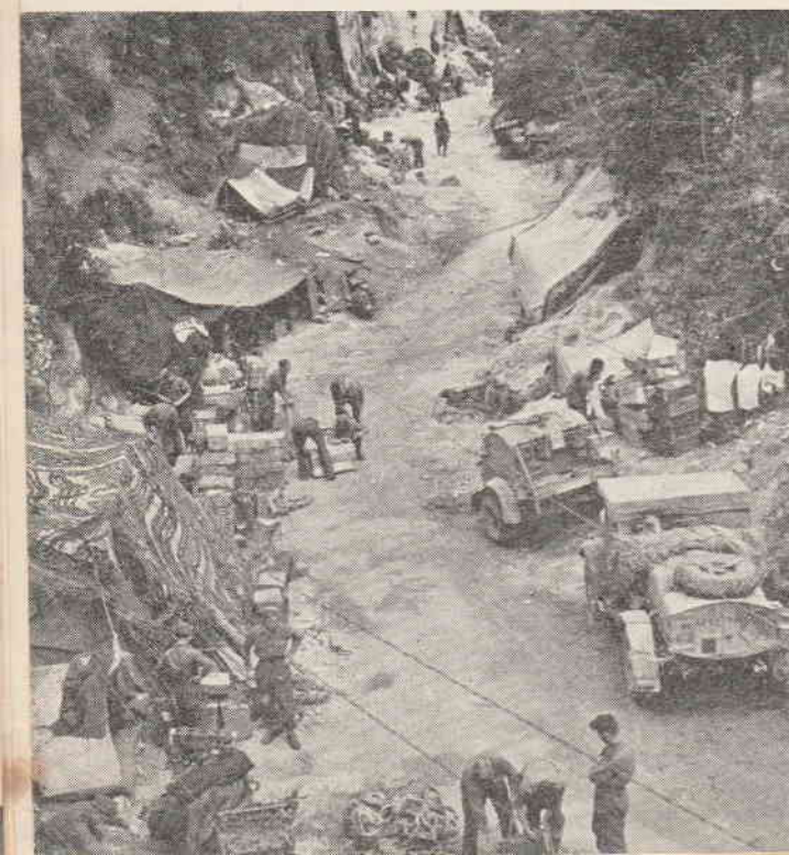
A SECTION OF THE HOVE DUMP
